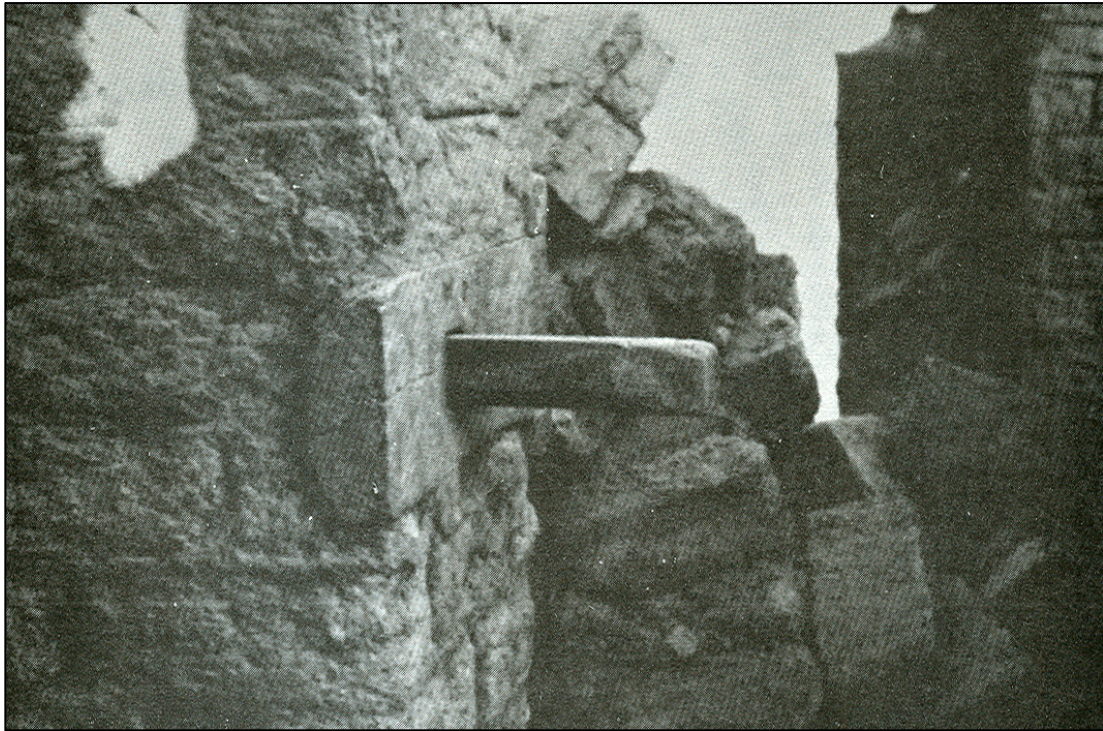
Figure 69: Wooden bolt for slide lock in its doorway casing at Karanis. Husselman 1979, pl. 48.
